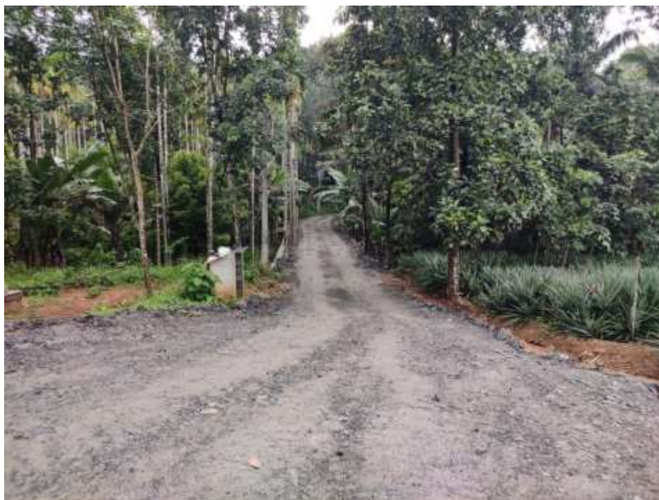
Figure 8: Photograph of Widened Access Road to Quarry
