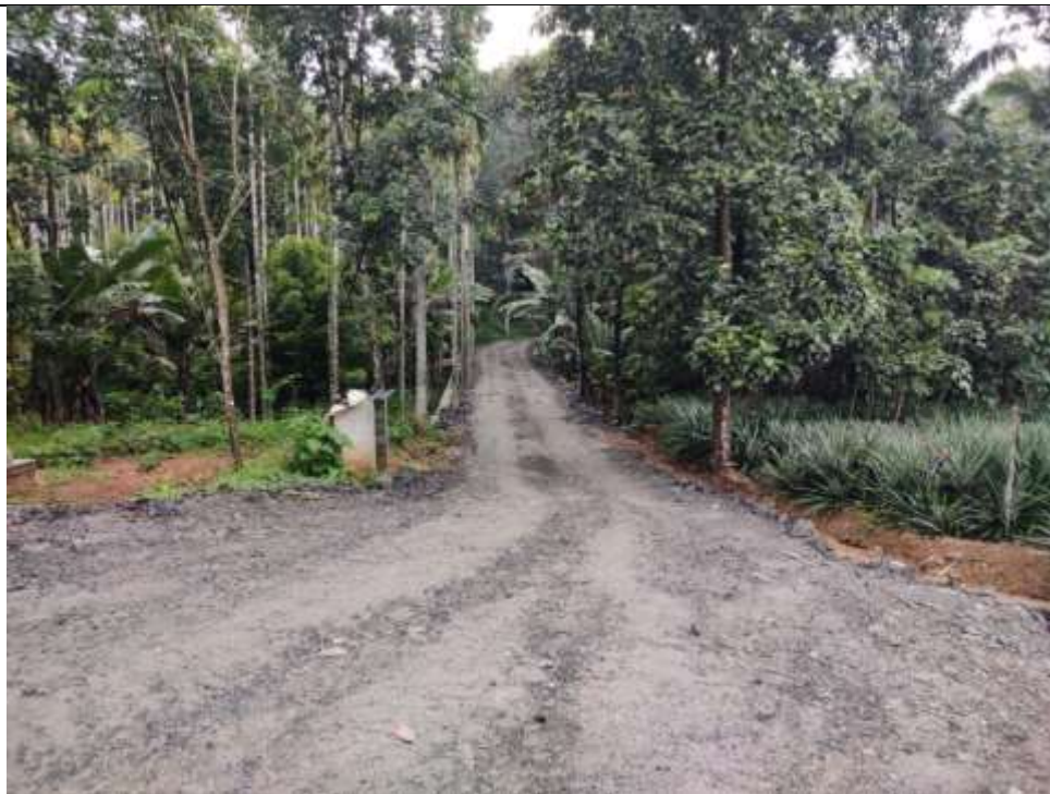
Figure 5: Photograph of Access Road to Quarry
