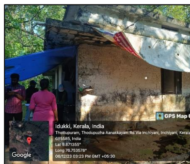
(262 m from BP 1) House of Mr. Raju Areekuzhiyil House No. 206 Ward No. 11
